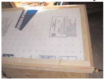
Detail showing how the 1 x 3 wood is attached outside the frame to eliminate drafts.
