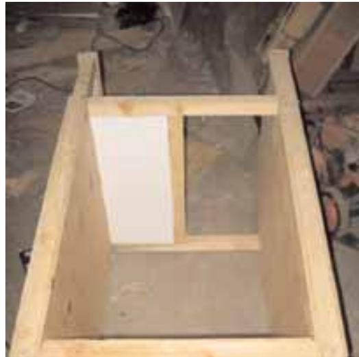
Only half of the front wall is open. The other half is insulated with polystyrene.
