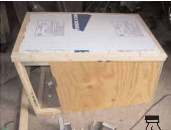
Roof likewise is filled with polystyrene.
